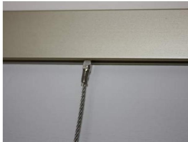
"T" head inserted into rail
